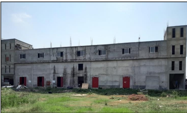
Building-2 (Utility Building)
