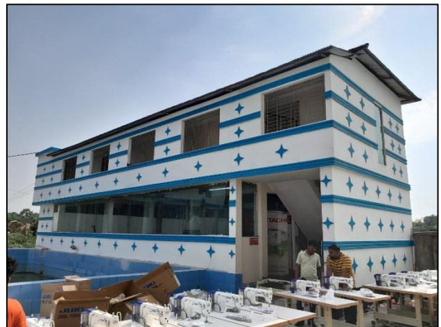
Building-3 (Fire Control Building)
