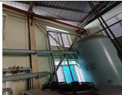
The thickness of wall bracing was found 5.3 mm instead of 6 mm
