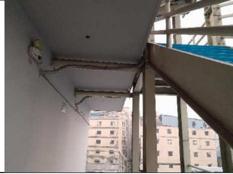
External Steel stair connected with Medical & daycare building.
