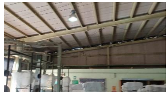
No compression strut in the long direction
