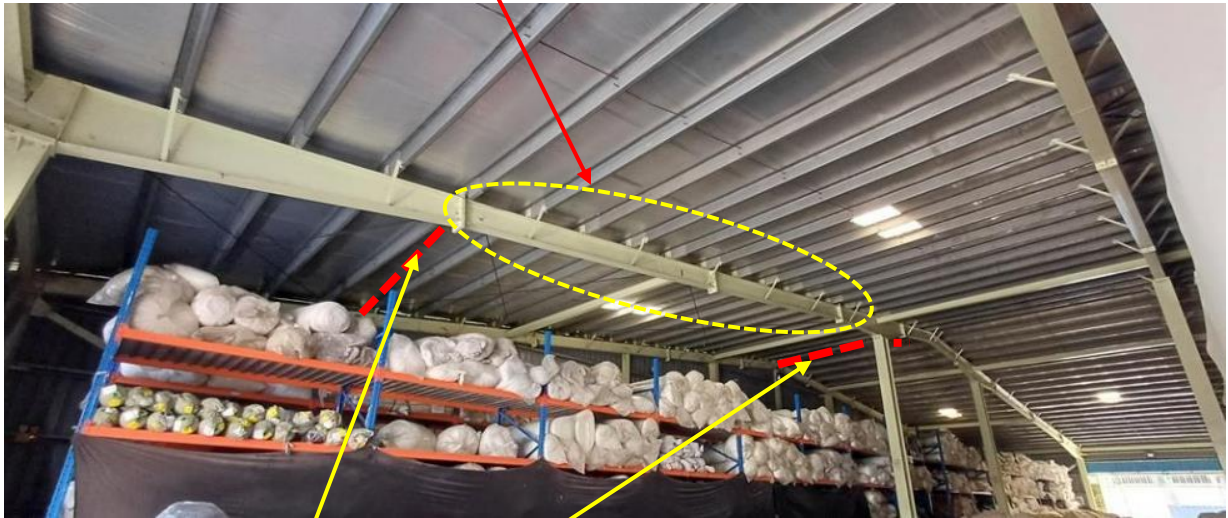
Proposed retrofitting on rafter in interior grid
