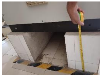
Floor buildup below LT panels at 1 st floor
