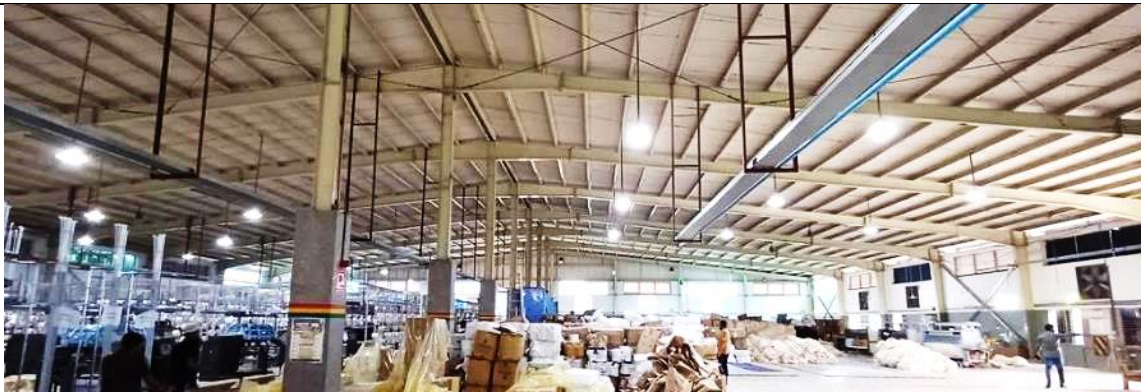
No compression strut in the long direction
