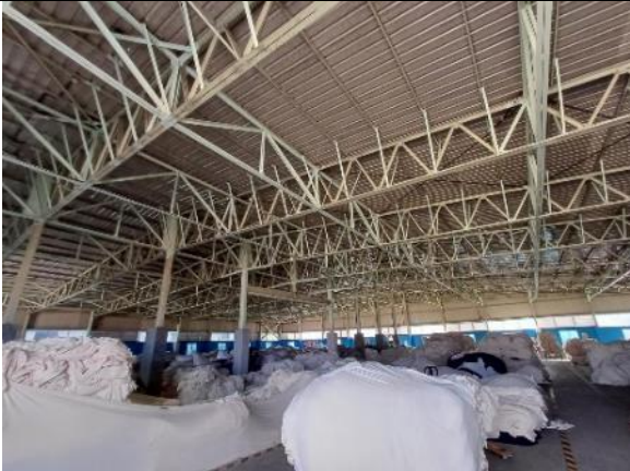
Steel truss along both directions
