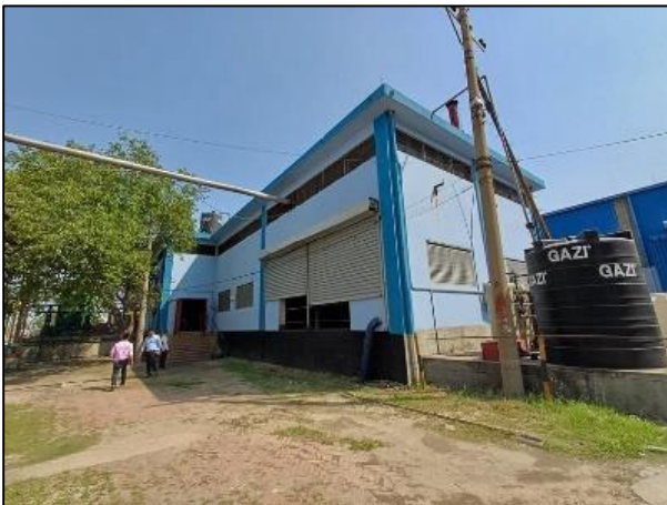
AOP Utility Building
