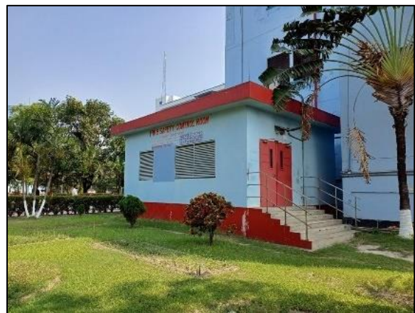
Fire Control Room
