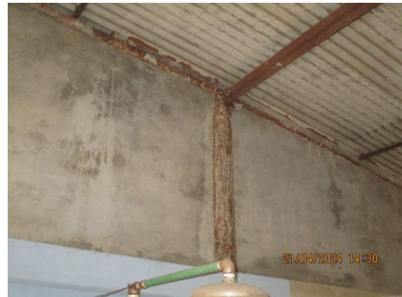
Chemical store shed
