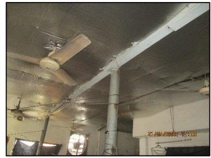
Ansar camp shed
