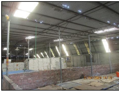
Wastage warehouse shed
