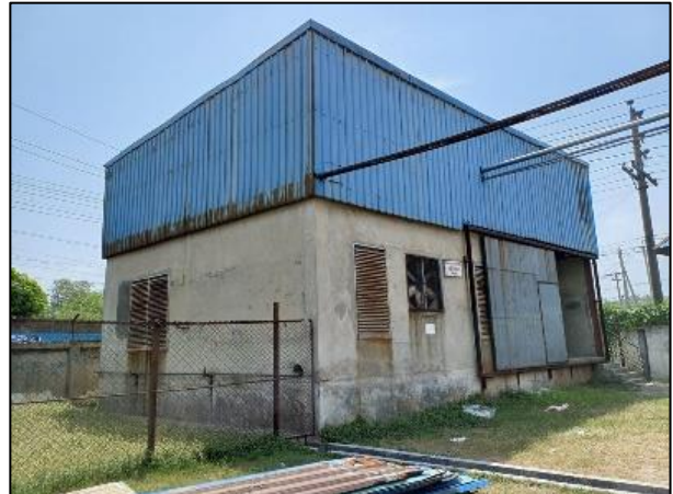
Jhut Boiler Room
