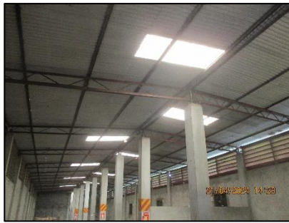
Chemical store shed
