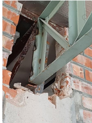
Roof truss to wall connection
