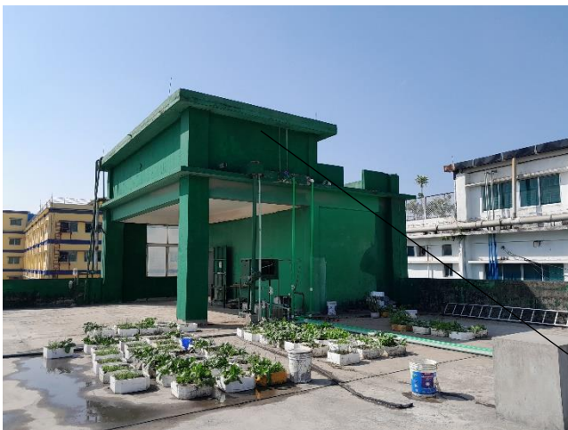
Onsite RC Overhead Water Tank
