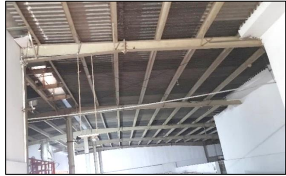
Finished goods store
