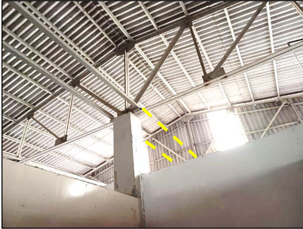
Discontinuous bracing (Shed 5)
