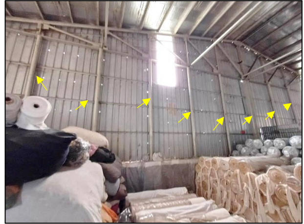
Additional pipe columns (Shed-10)
