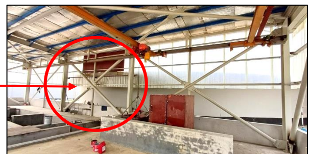
Additional pipe columns (Shed-10)
