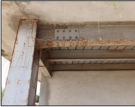
Corrosion at main beam
