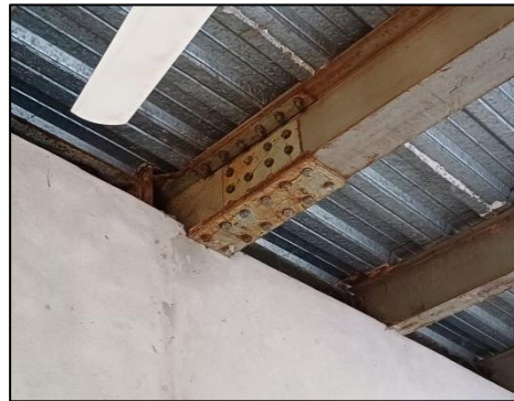
Corrosion at stair
