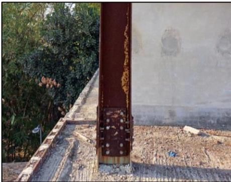
Corrosion at main beam
