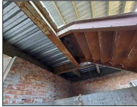
Corrosion at stair
