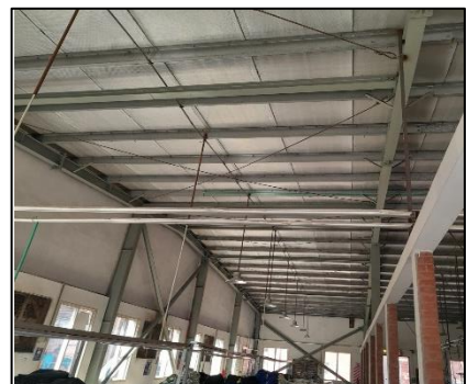
Missing bracing
