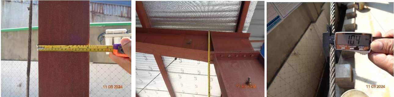
Flange thickness of SC1, SC2 and SC3 (from left)
