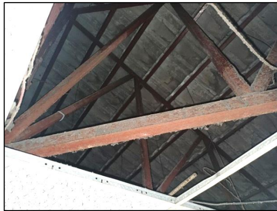
Steel roof top shed
