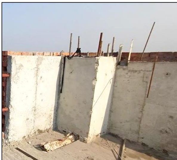
Exposed Rebar
