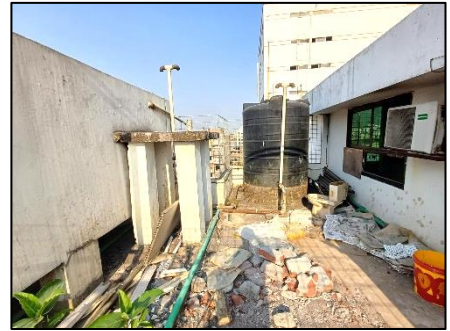
PVC water tank at the roof
