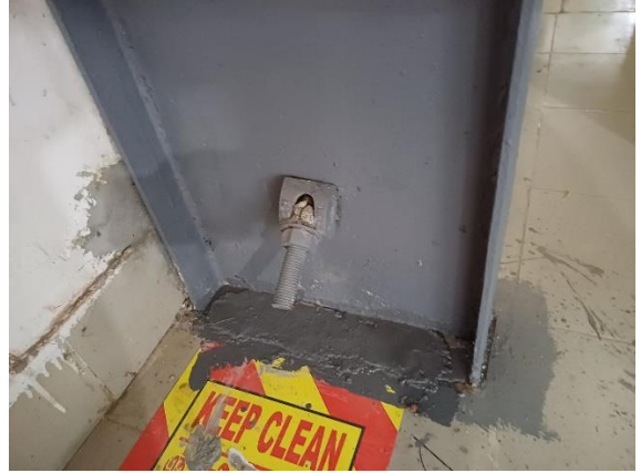
Connection of deformed bar
