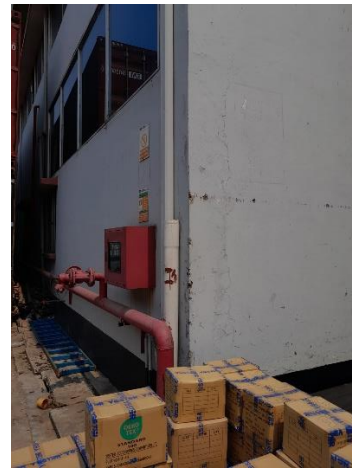
Button injection building
