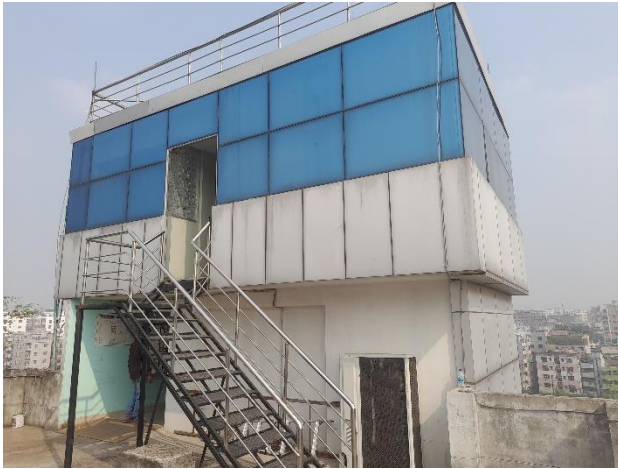
Rooftop RC structure
