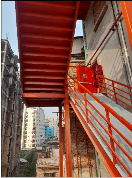
External steel stair without any vertical and horizontal bracing
