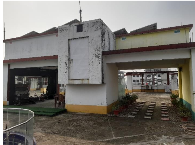
Rooftop RC O.W.R
