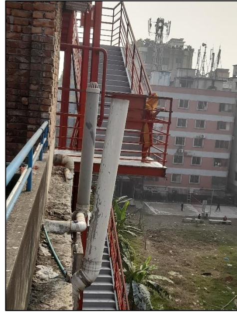
External steel stair without any vertical and horizontal bracing
