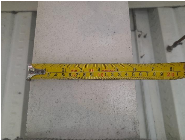
Main beam flange size measured 150 mm
