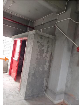
Additional 250mm wall for fire door.
