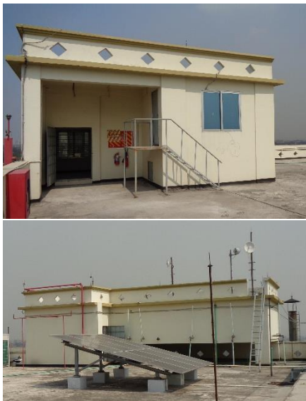
Staircase and OHWT
