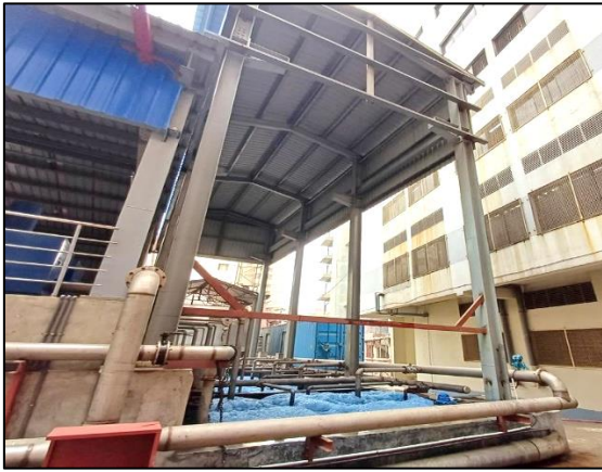
No bracing (Shed 2)
