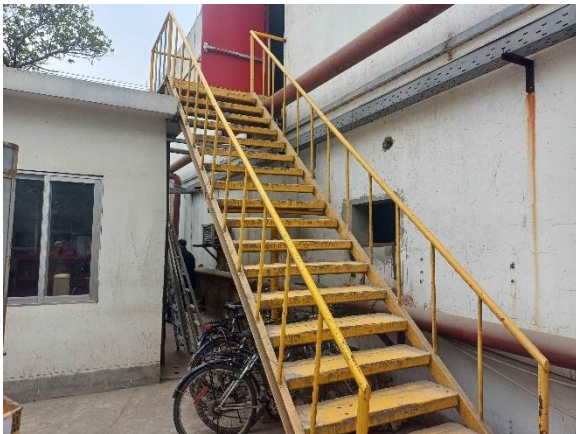
Apparently non-engineered steel stair
