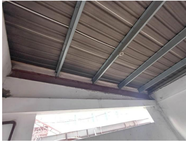
No load transfer media at long-direction
