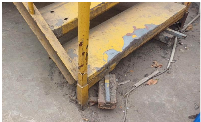
Apparently non-engineered steel stair
