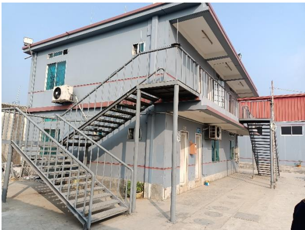
External steel stair
