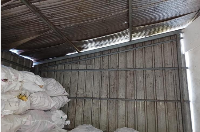
Steel angle connection with steel column
