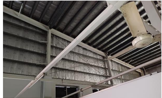
Compression strut on end bay
