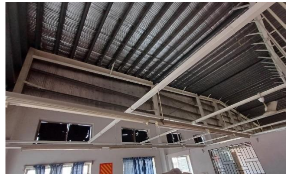
Compression strut on end bay
