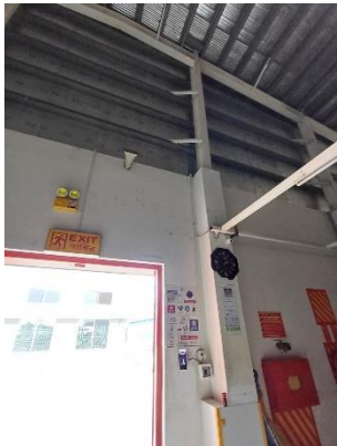
Incline column at East
