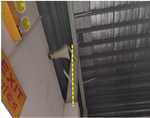
Incline steel column
