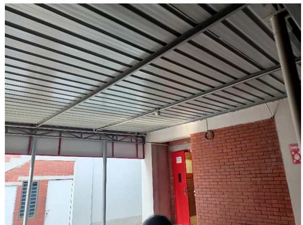
Truss and column frame
