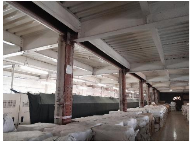
Steel framing systme
