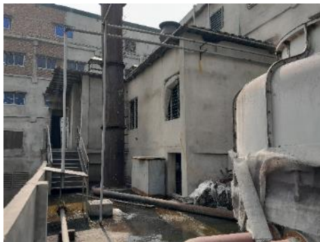
Undocumented roof top shed
