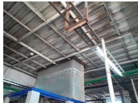
Apparently non engineered roof shed
