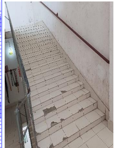
South Stair: numbers of tread, height of riser, and landing width are mismatching with provided drawing
