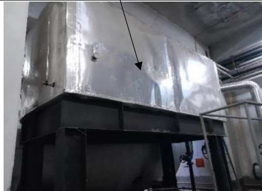
Missing RC column.
