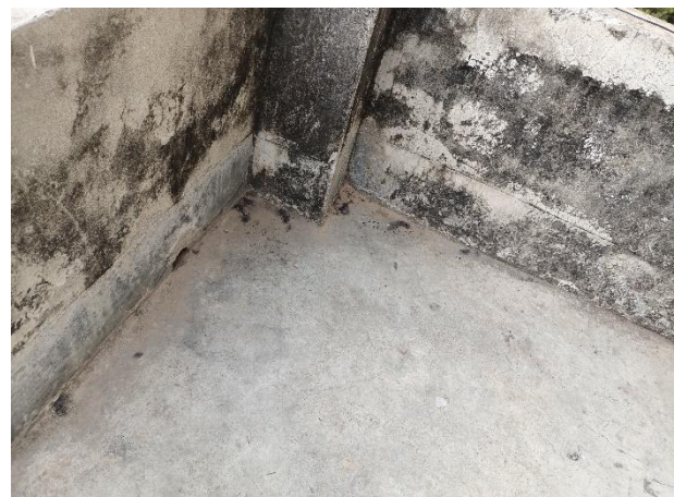
Parapet on roof
