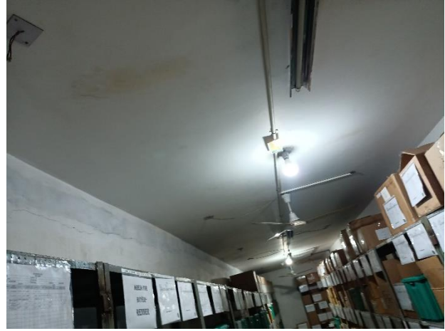
Unbraced racks on floor
