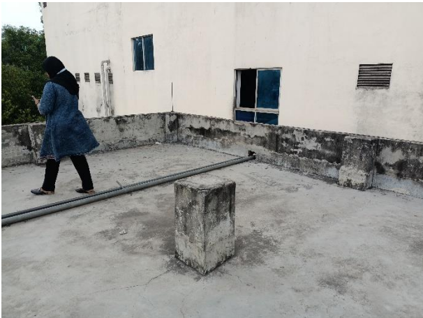
Parapet on roof
