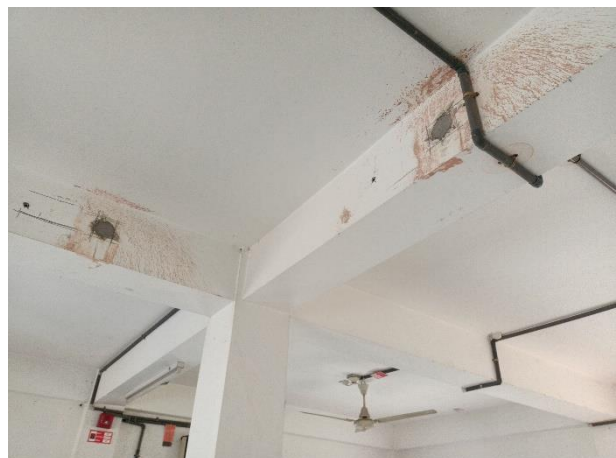
Core cutting location
