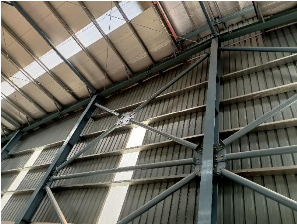
Vertical bracing and compression strut
