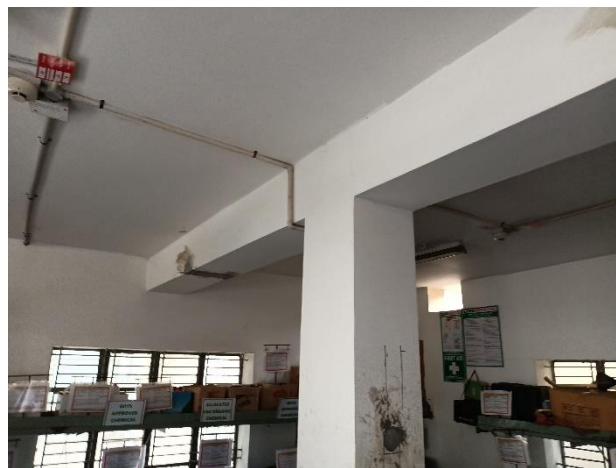
Core cutting location
