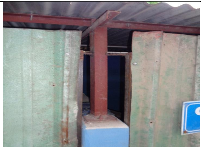
Connections of angle 'L'
