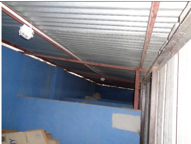
MS angle supported lightweight steel roof
