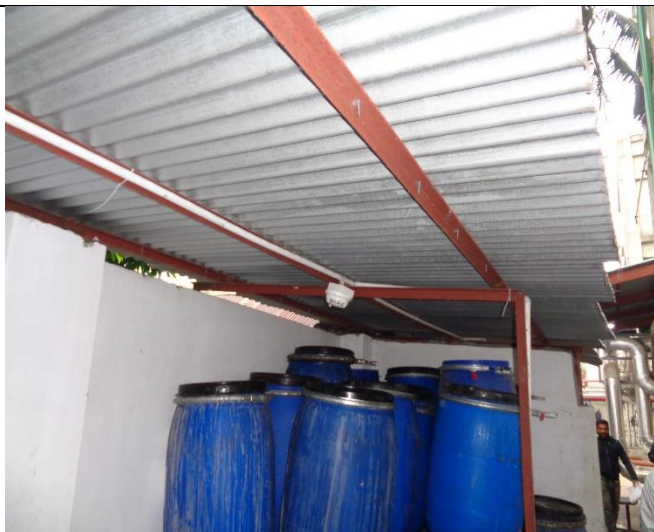
MS angle supported lightweight steel roof
