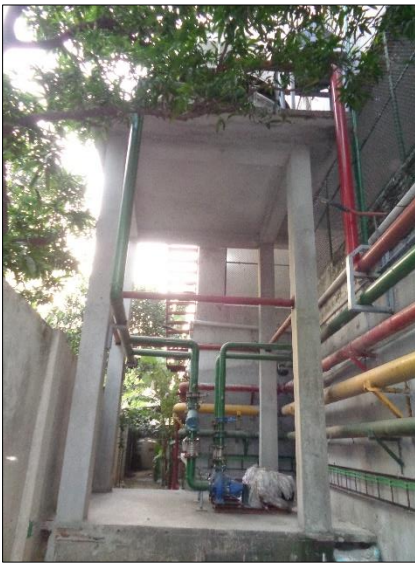
Cooling Tower Building-2
