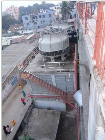
Cooling Tower Building-4
