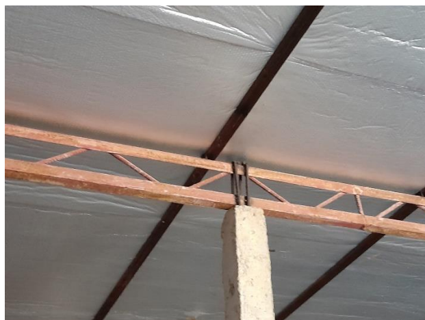
Poor Connection
