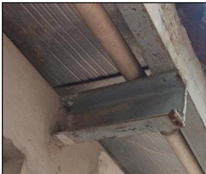
Rafter inserted to brick wall connection (Daycare Shed)
