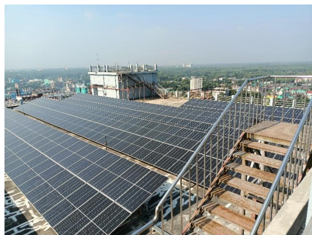
Steel stair on the roof
