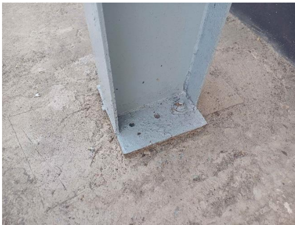
Bolt missing found in several locations
