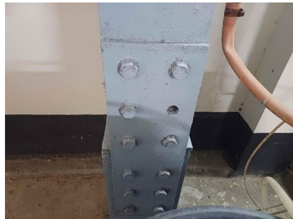
Bolt missing found in several locations
