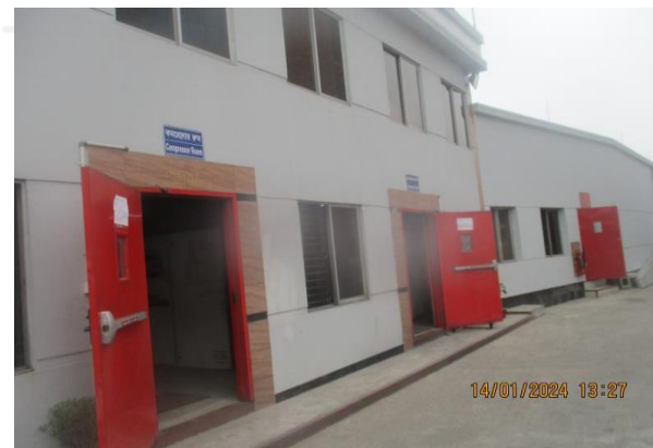
Building No.: 3; (Security Post & Sub-station Building, Partially G+1, RCC Building).
