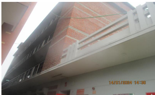
Building No.: 2; (Officers Resting Room, B+G+3, RCC Building).
