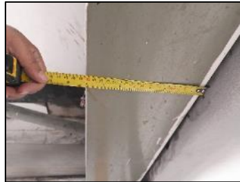
Steel column SC1 found instead of SC3. (At 2 nd floor) (280x550) mm
