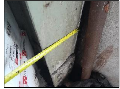
Steel column SC3 found (200x400) mm instead of (200x260) mm. (At 2 nd floor)
