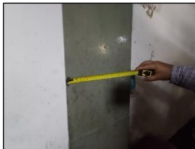
Steel column SC2 found instead of SC1. (At 2 nd floor)
