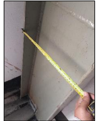
Steel column SC3 found (200x400) mm instead of (200x260) mm. (At 2 nd floor)
