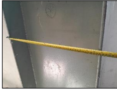
Steel column SC1 found instead of SC3. (At 2 nd floor) (280x550) mm
