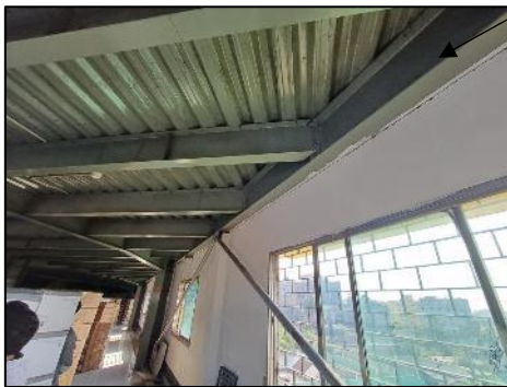
Marked beam details not shown in drawing (180x400) mm
