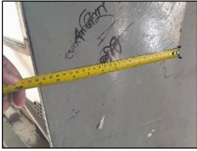
Steel column SC1 found instead of SC3. (At 2 nd floor) (280x550) mm
