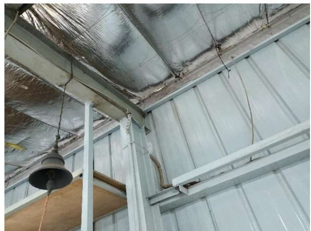
No load transfer media is provided along long direction
