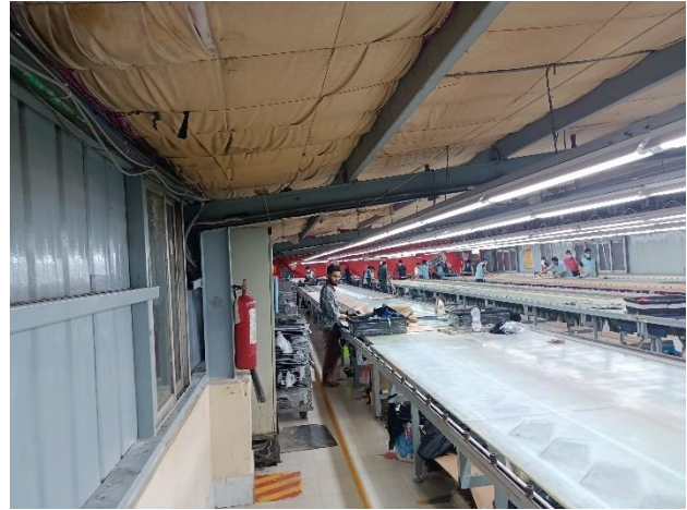
Framing of Printing Shed
