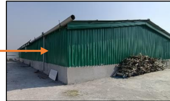
Undocumented Roof Shed
