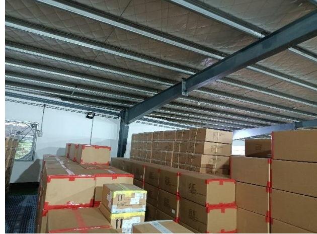
Framing of 116 Finished Goods Shed
