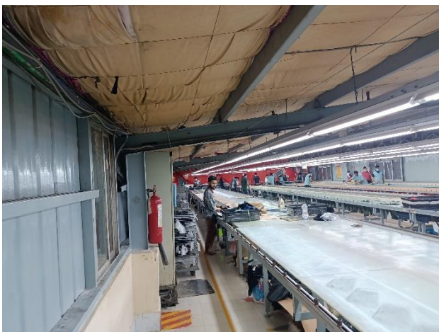
No load transfer media is provided along long direction
