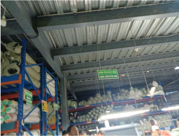
Beam-column of mezzanine
