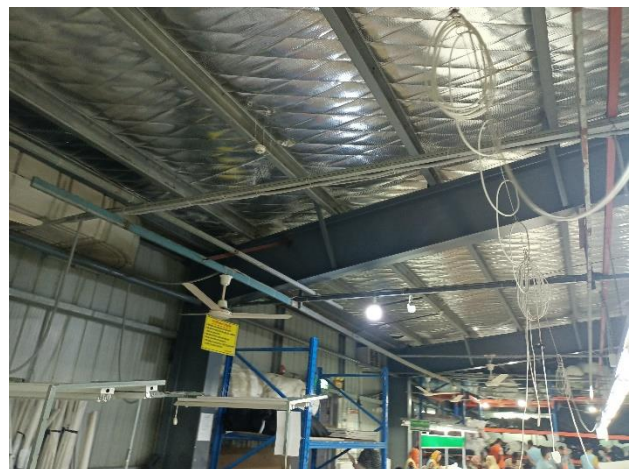
Framing of roof
