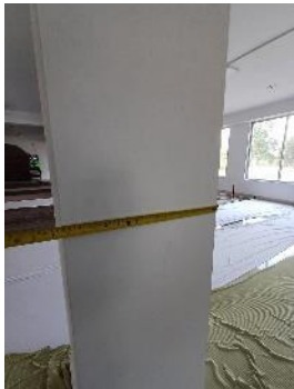
Mismatch in column size at column schedule
