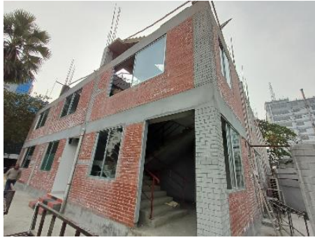
Building 3 constructed up to 2 storey
