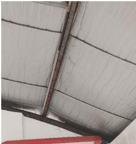
Severe corrosion on steel members
