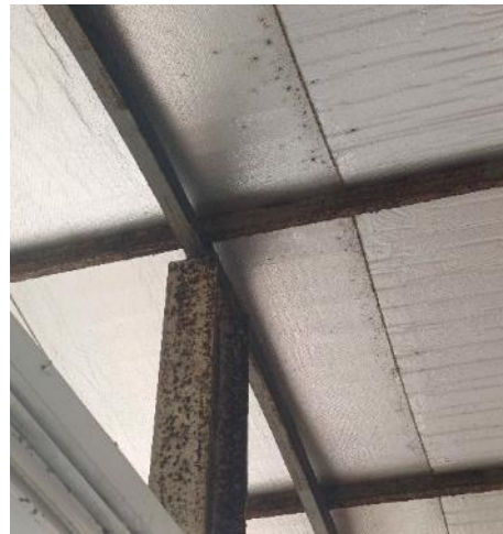
Severe corrosion on steel members
