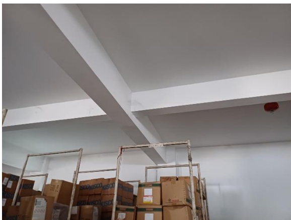
Beam offset from column center
