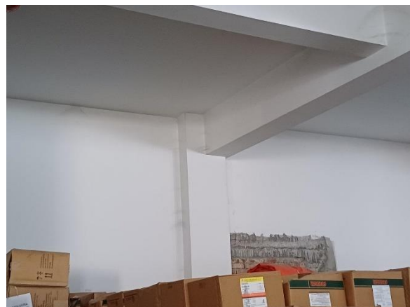
Beam offset from column center
