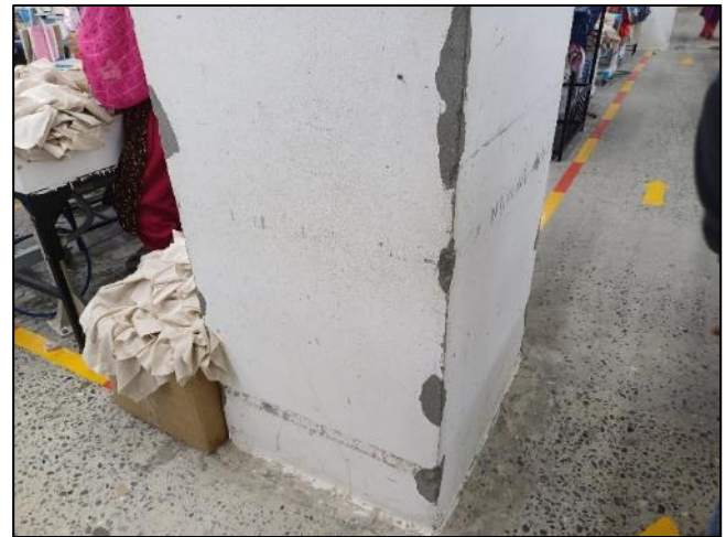
Trolley impact on column
