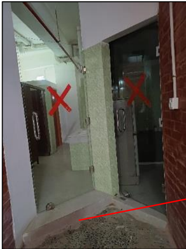
150 mm build-up found at the toilet zone of 1 st floor which is not mentioned in the drawing.
