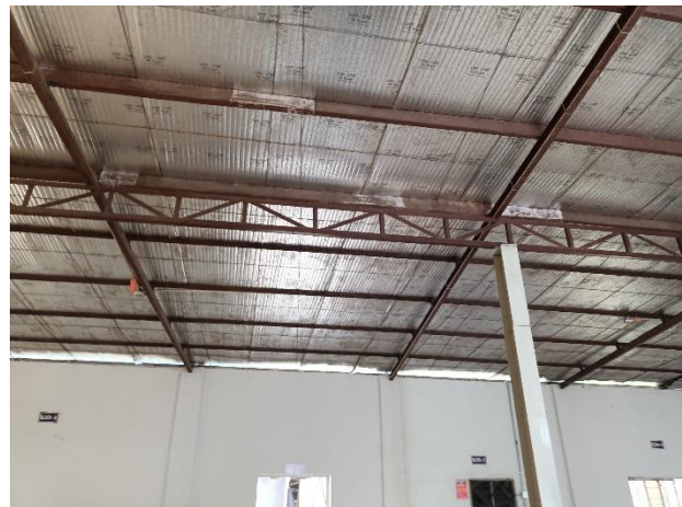
Steel angle connected with brick walls
