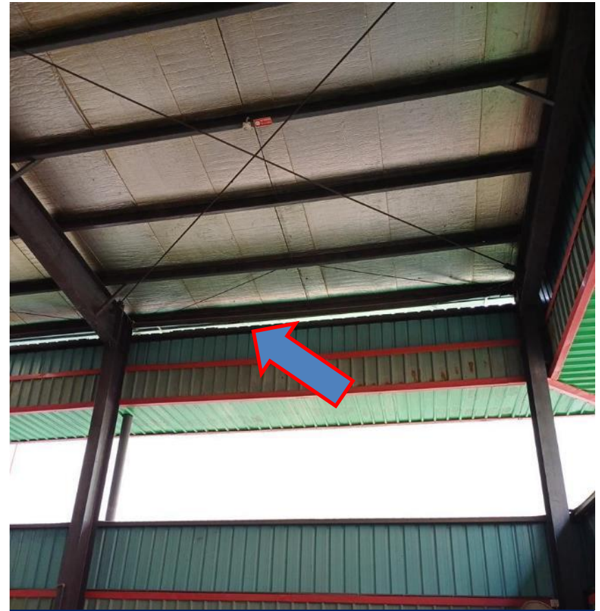
Only roof bracing and compression member
