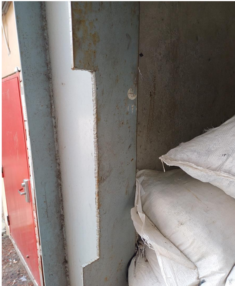
Sample has been taken from Column Flange
