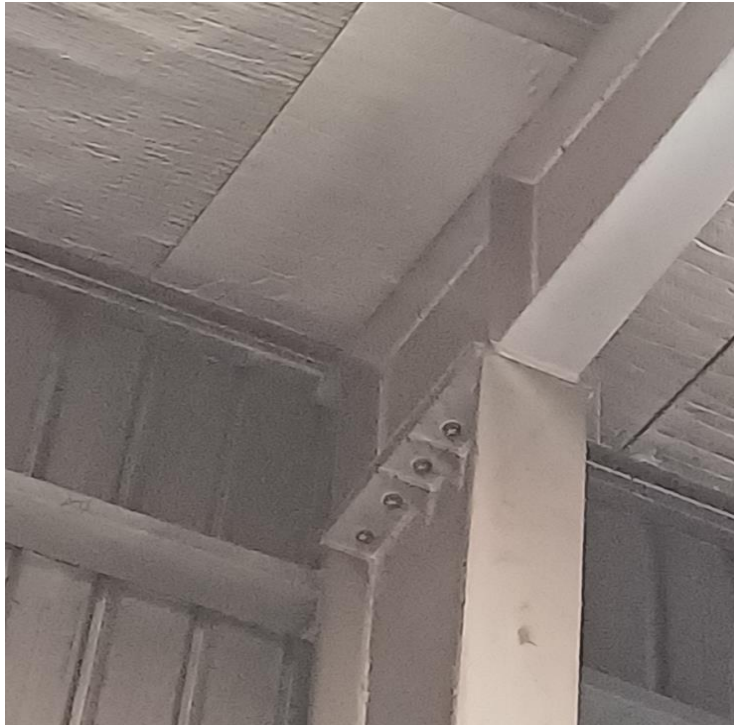
column-rafter connection
