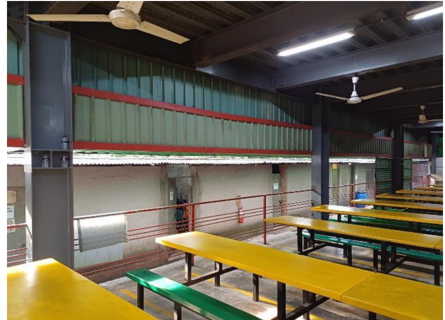
Columns found in transverse direction
