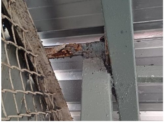
Severe corrosion at steel member
