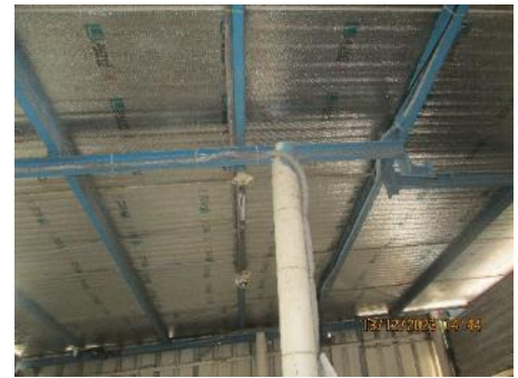
Loading & unloading shed of WP
