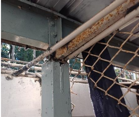
Severe corrosion at steel member
