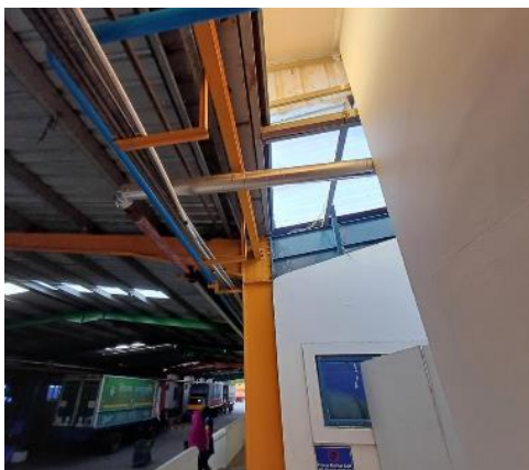
Canteen Building and Rain Protection shed – Structurally Connected
