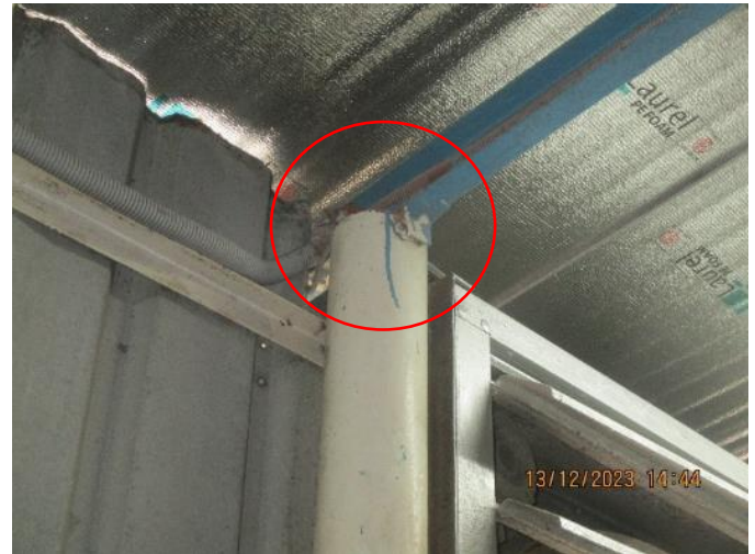
Loading & unloading shed of WP
