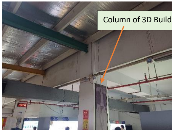
Structurally Connected Column
