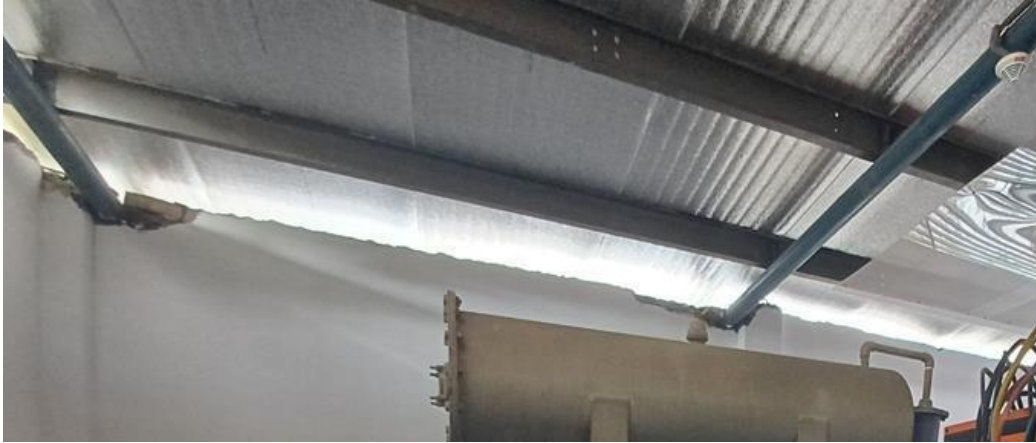
Connection between pipe and brick wall
