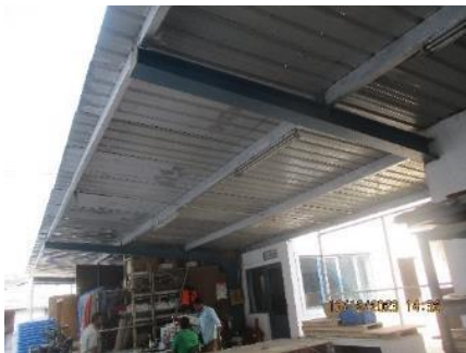
Maintenance workshop shed
