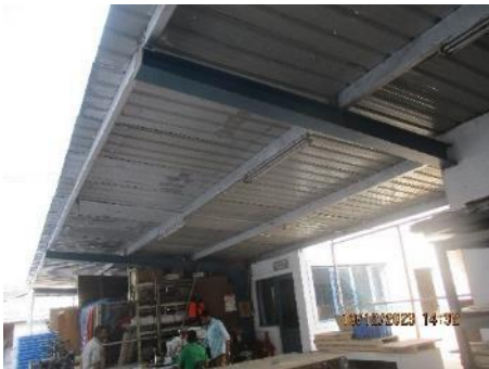
Maintenance workshop shed
