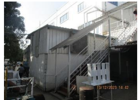
Loading & unloading shed of WP
