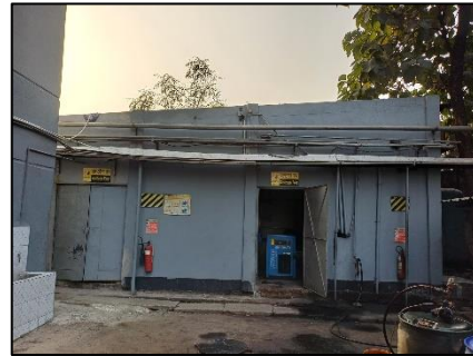
Shed 5-Substation Shed
