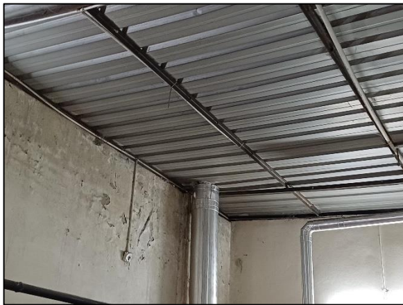
Shed 6-Compressor Shed
