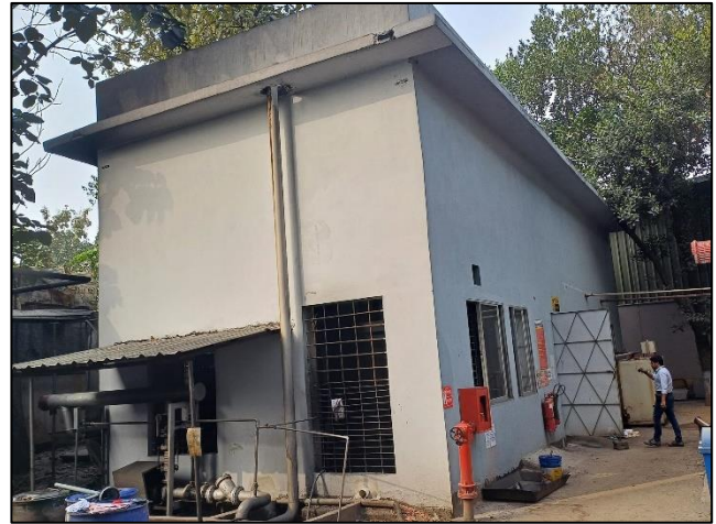
Building 2-Generator Building
