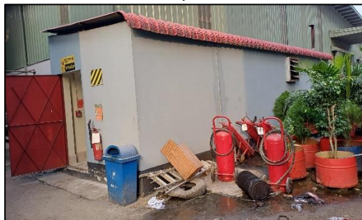
Shed 8-Fire Pump Shed
