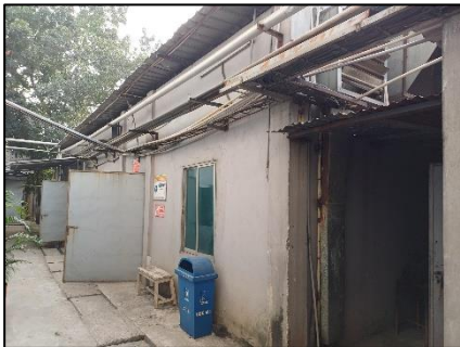
Shed 6-Compressor Shed
