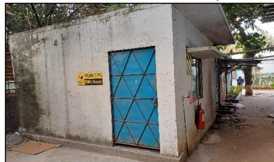
Building 3-RMS room
