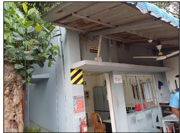
Shed 7-Fire Control & Security Shed
