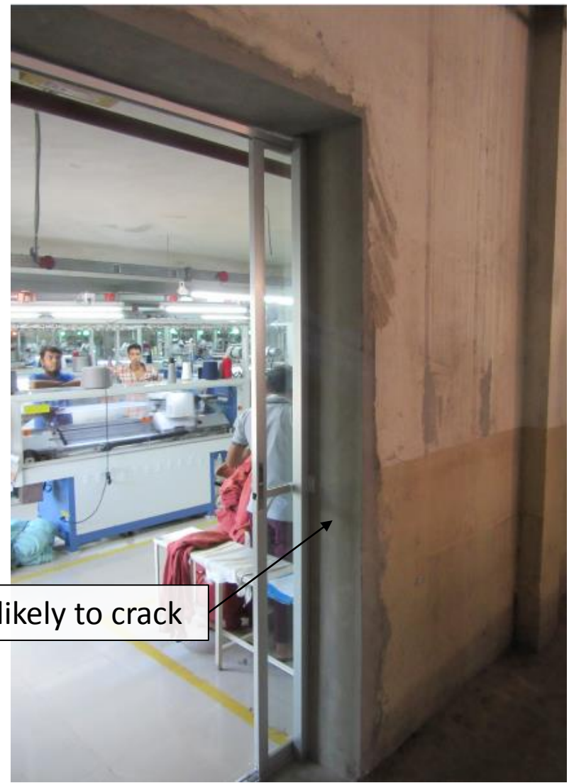
The joint between factory building and existing shed has been plastered over
