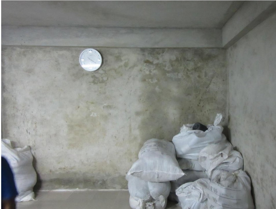
Damp observed on ground floor at East end of building
