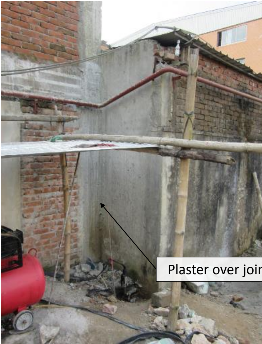
The joint between factory building and existing shed has been plastered over
