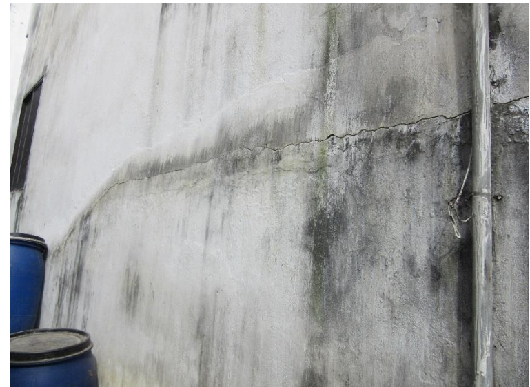
East Facade - Ground Floor
