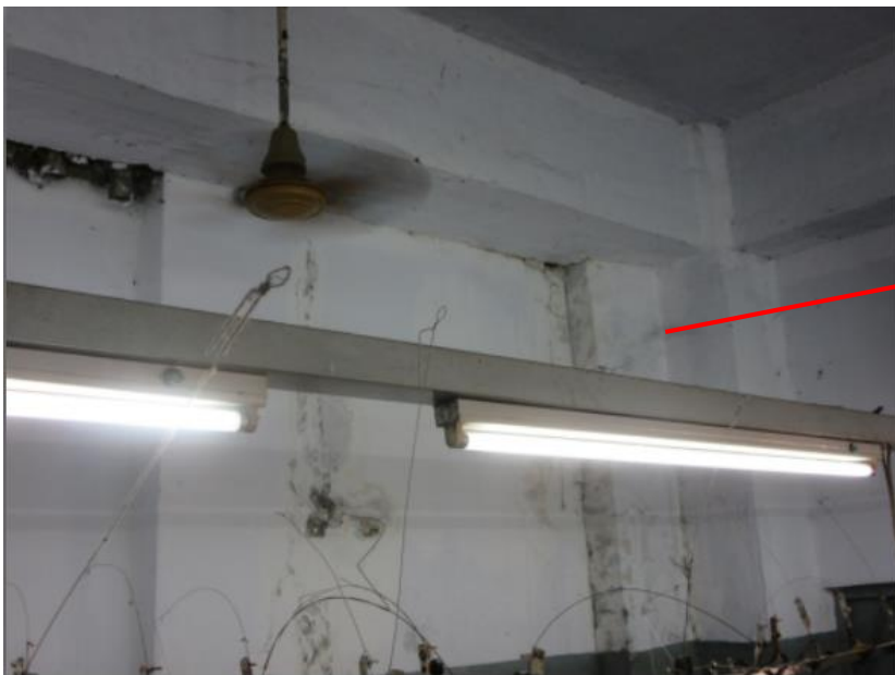
Standing water on the roof
