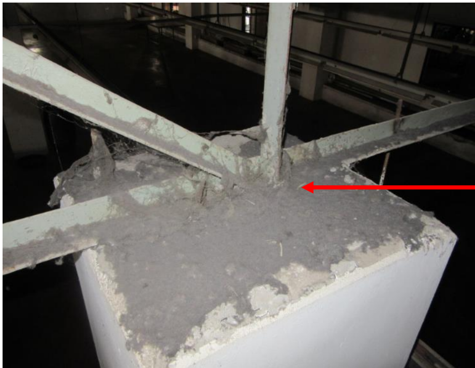
Non-engineered connections
