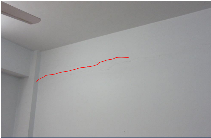
1st Floor. Horizontal crack on the partition walls
