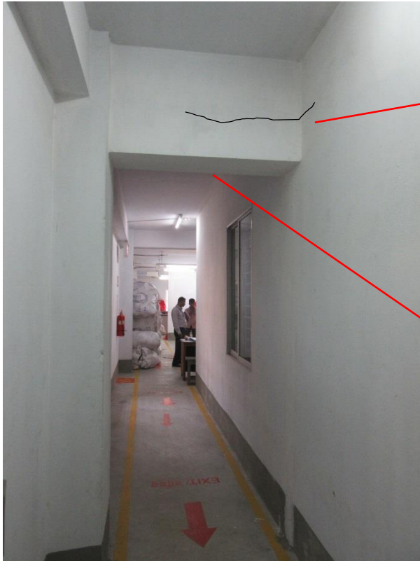
2nd Floor. Horizontal crack on the beam
