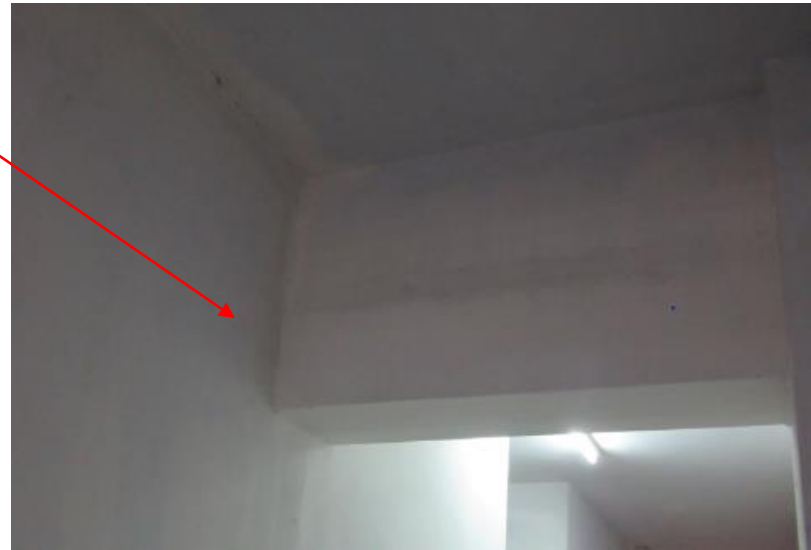
2nd Floor. Horizontal crack on the beam
