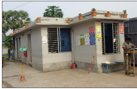
Security & RMS Room
