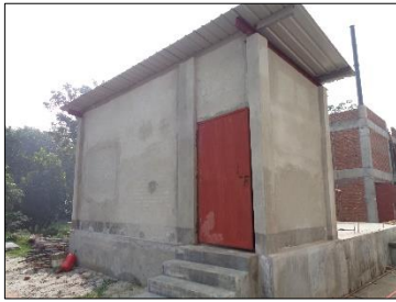
Fire Pump Room
