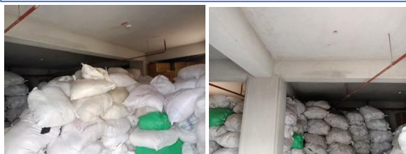
Roof floor loading
