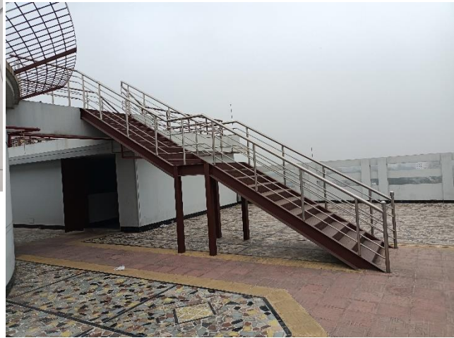
Steel stair on roof
