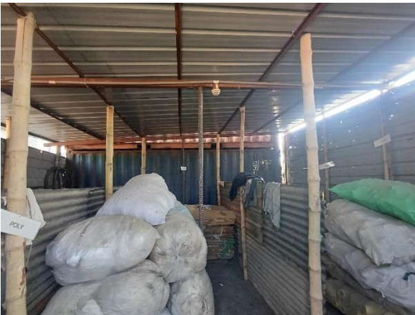
Apparently non-engineered shed (supported on bamboo)
