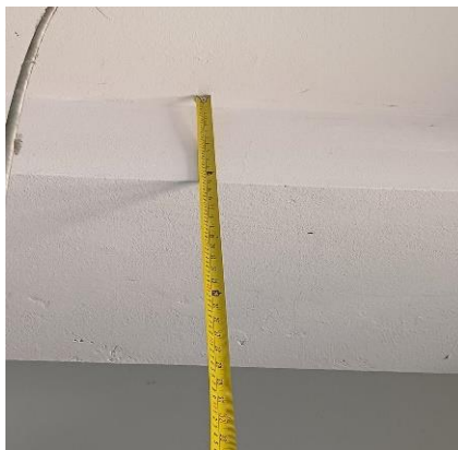
Mismatches in floor beam sizes
