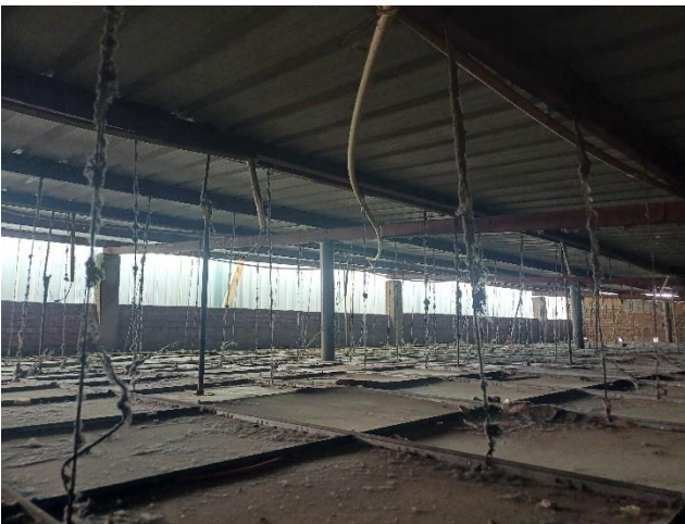
Absence of load transfer media (Strut & bracings) along long directions & improper connections
