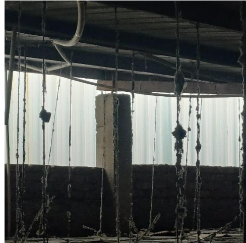
Absence of load transfer media (Strut & bracings) along long directions & improper connections
