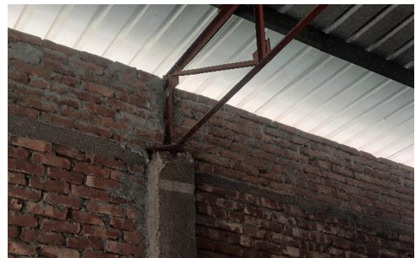
Absence of load transfer media (Strut & bracings) along long directions & improper connections
