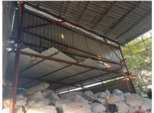
Absence of load transfer media (Strut & bracings) along long direction
