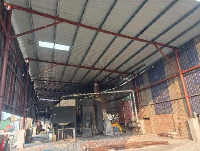
Absence of load transfer media (Strut & bracings) along long direction
