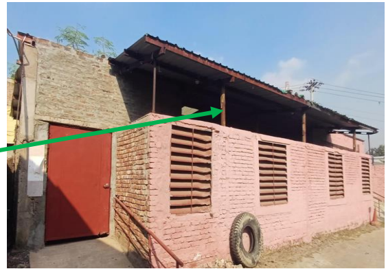
Steel column not shown in as-built drawing
