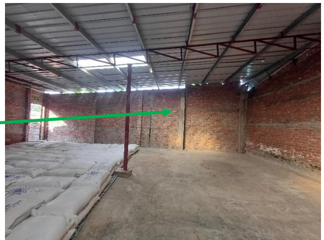
RCC column location not matched in as-built drawing
