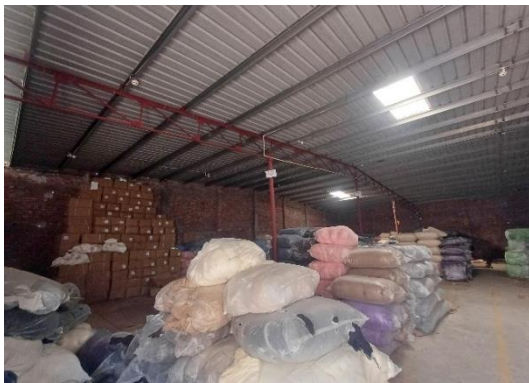
Absence of load transfer media (Strut & bracings) along long directions & improper connections
