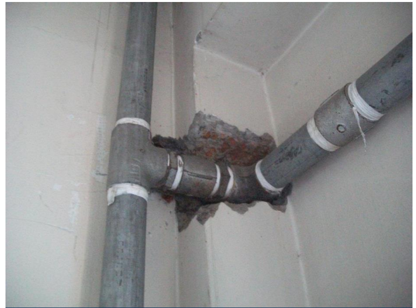
A significant portion of column has been removed, possibly cutting rebar.
