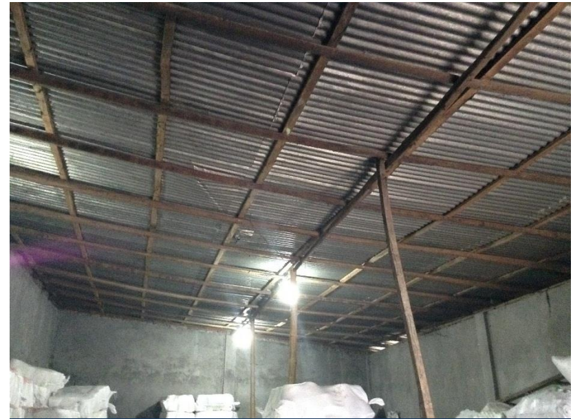
Non-engineered wooden framing of Generator/Storage building
