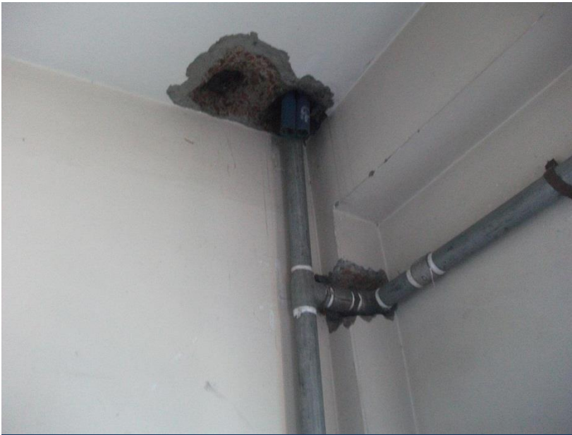
Services chased through slab
