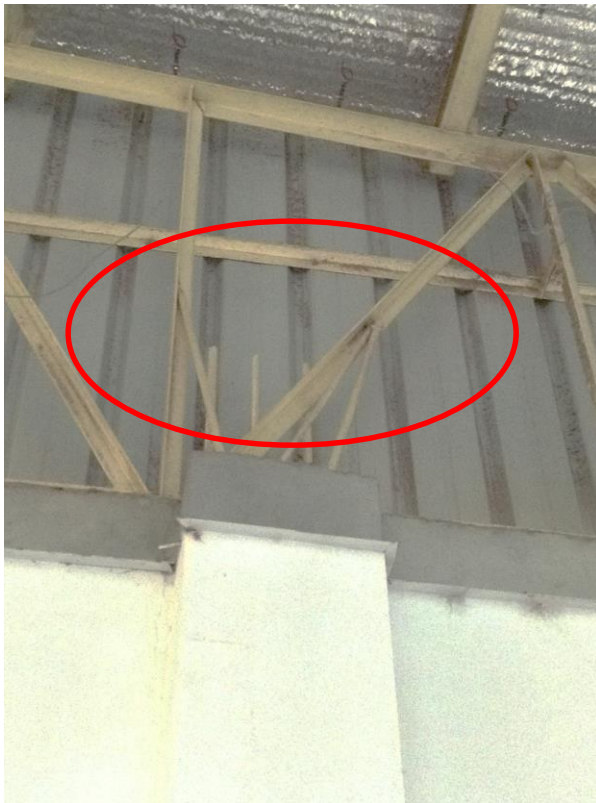
Truss resting on top of the RC columns welded to column rebars
