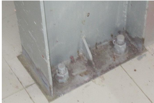
Typical end plate detail of internal column
