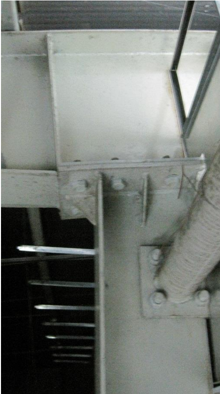
Top plate detail – semi rigid flexible connection
