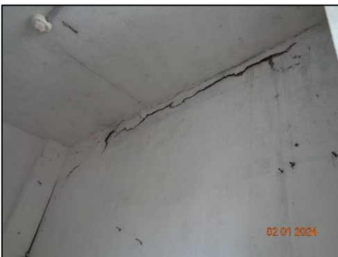
Sludge storage room
