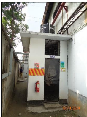
Sludge Storage Room
