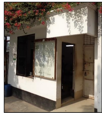
Access Control Room
