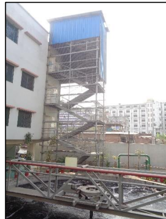
Stair at west side
