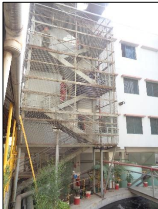
Stair at east side
