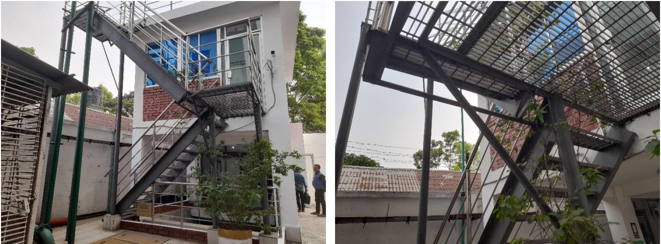
Inadequate connection
