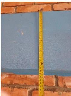
Tie Beam Size found. (300mm X 300mm)
