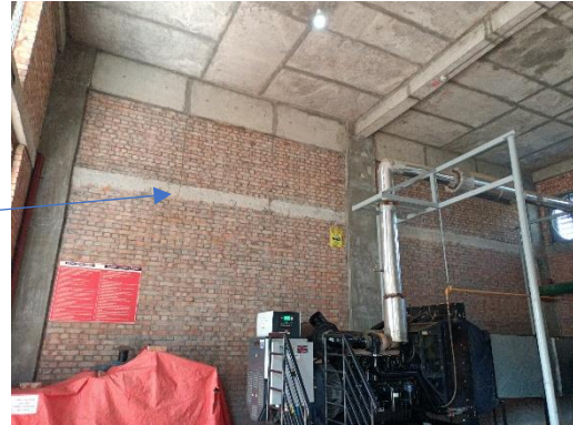
Tie beam on site
