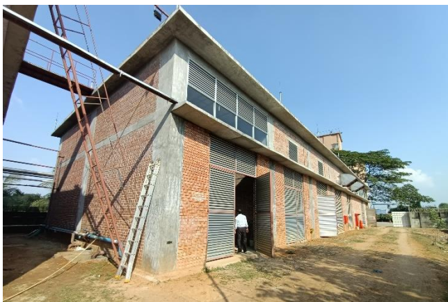
Substation & Generator Building
