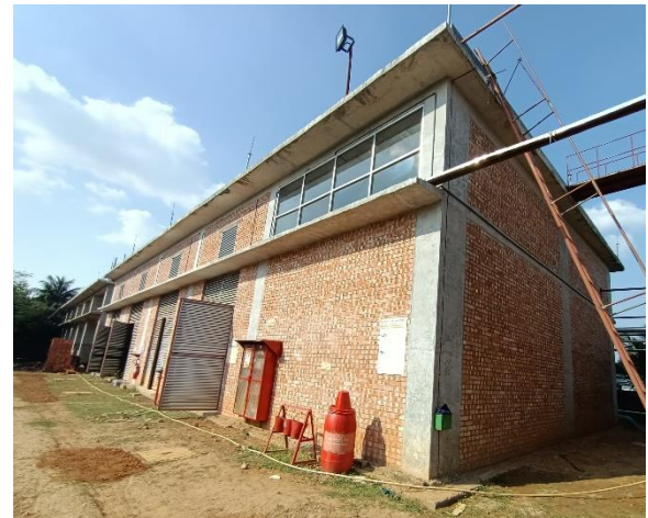
Boiler & Compressor Building
