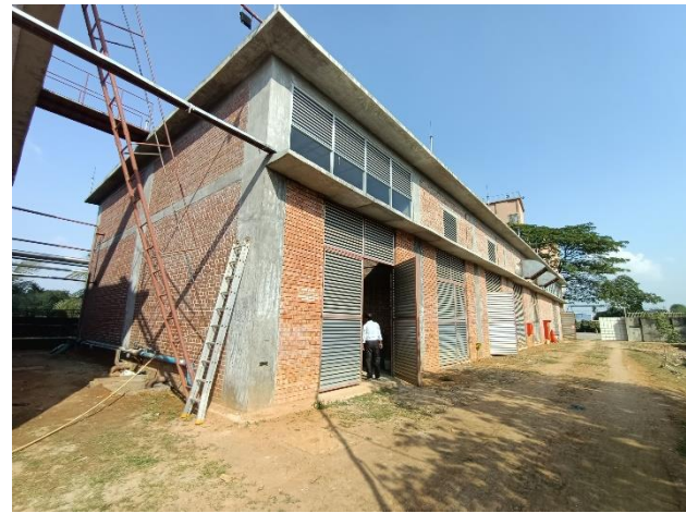
Substation & Generator Building
