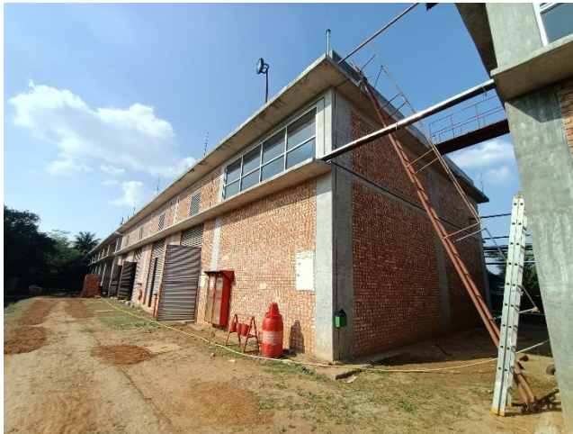
External Steel stair/ladder
