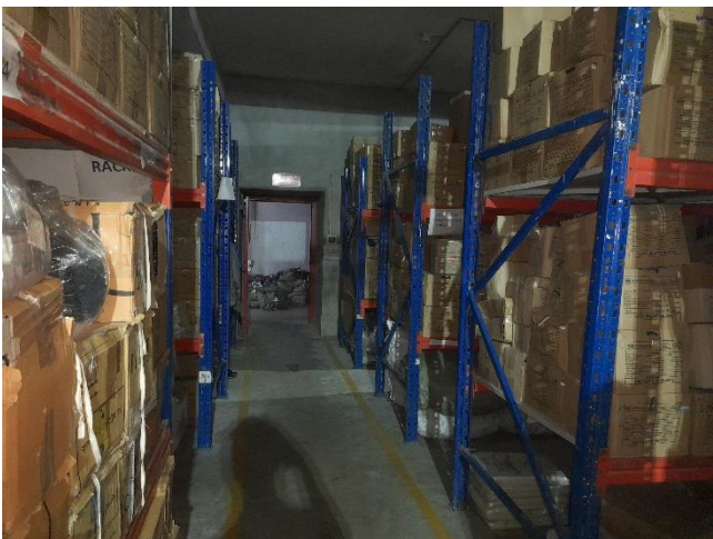
Unbraced storage racks on floors
