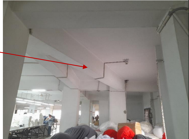
Roop top beam slab level
